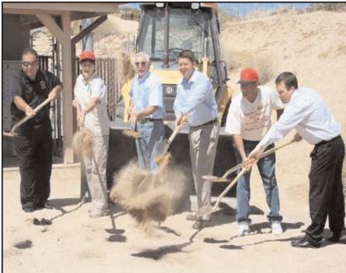
Prominent supporters of the Jawbone Station break ground for its expansion
